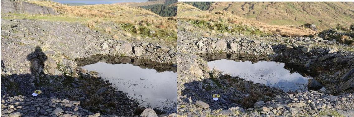
Plate 7.9: Turbine T02 Foundation Excavation
