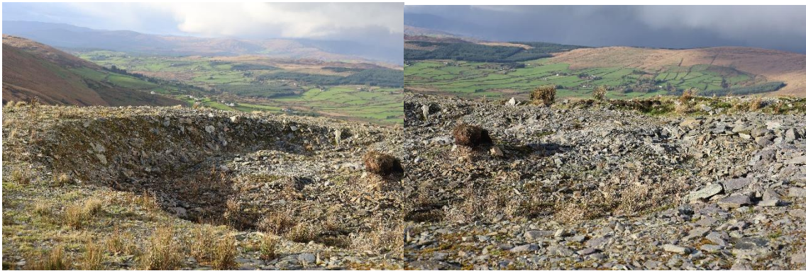
Plate 7.8: Turbine T01 Foundation Excavation
