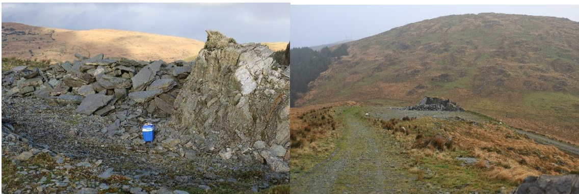
Plate 7.10: Turbine T03 Foundation Excavation
