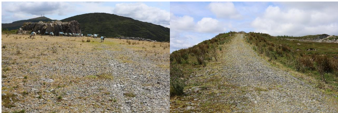
Plate 7.7: Wind Farm Access Roads
